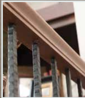
Iron Balusters Installed to handrail
