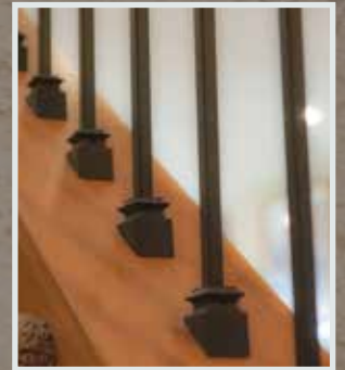
Iron Balusters Installed with pitch shoes
